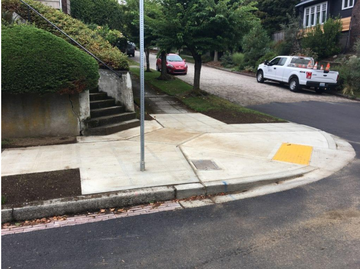
Figure 5: A curb ramp with truncated domes at E Valley Street and 24 th Avenue E in Seattle (Tupper, 2019)
